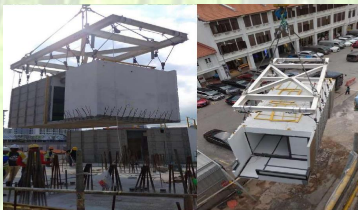
Photograph 7 - Prefabricated Prefinished Volumetric Construction (PPVC)
