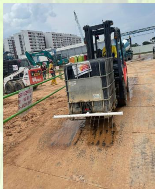
Photograph 4 – Ways on how recycled water from treatment plant are being used.
