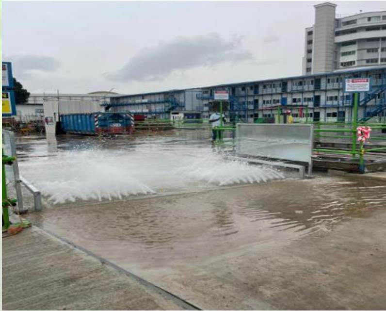
Photograph 3 – Auto water spraying system.
