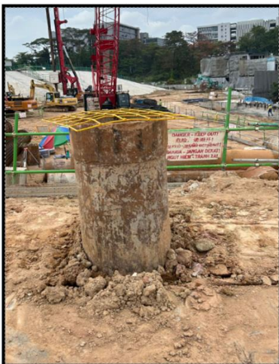
Scrap rebar reused to fabricate bore piling casing cover
