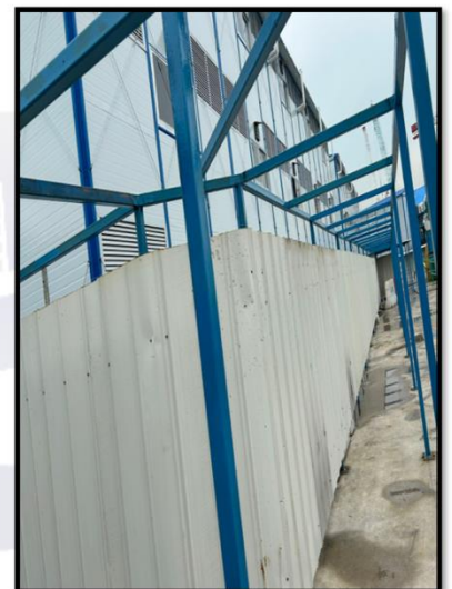
Scrap hollow section and zinc sheet reuse to construction overhead shelter and hoarding
