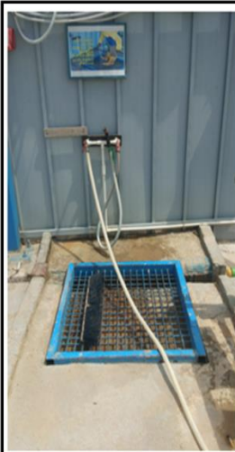
Tap Point with Spray Gun to ECM Pond Recycle Water Usage During Washing Boots
