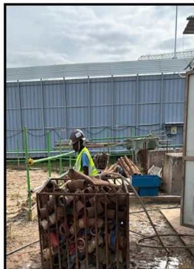
Scrap rebar reused to fabricate silo joint fitting rack
