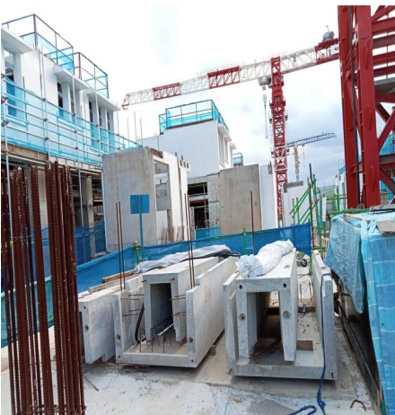
Use of Precast house drain
