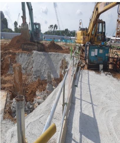
Reuse waste hardcore to slope earth protection
